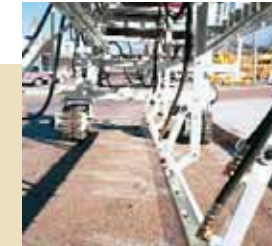
Longitudinal texturing with hydraulically adjustable comb pitch
