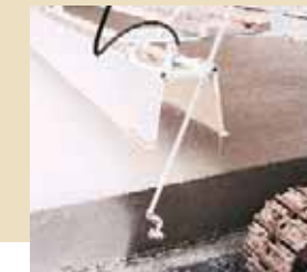
Adjustable longitudinal spray bar for concrete slab and side edge curing
